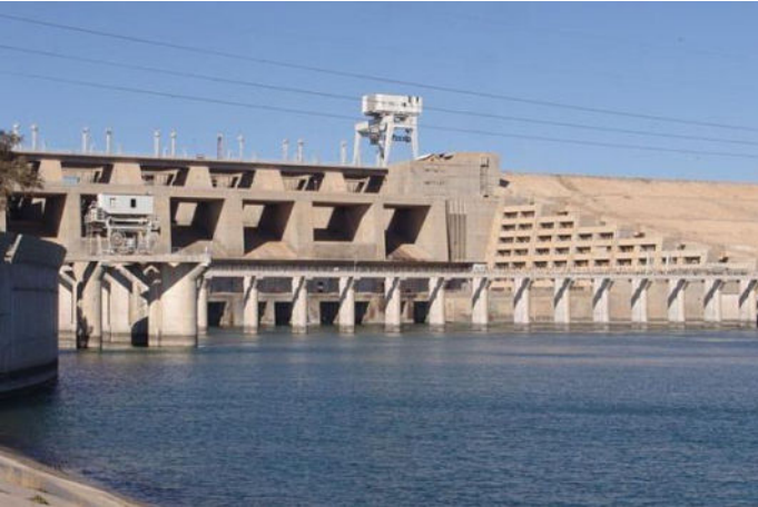
Haditha Dam is an earth-fill dam on the Euphrates, north of Haditha, Iraq
